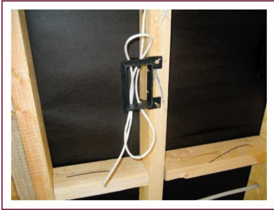
EXHIBIT 800.5 Communications outlet provision installed at "rough-in." (Courtesy of the International Association of Electrical Inspectors)
