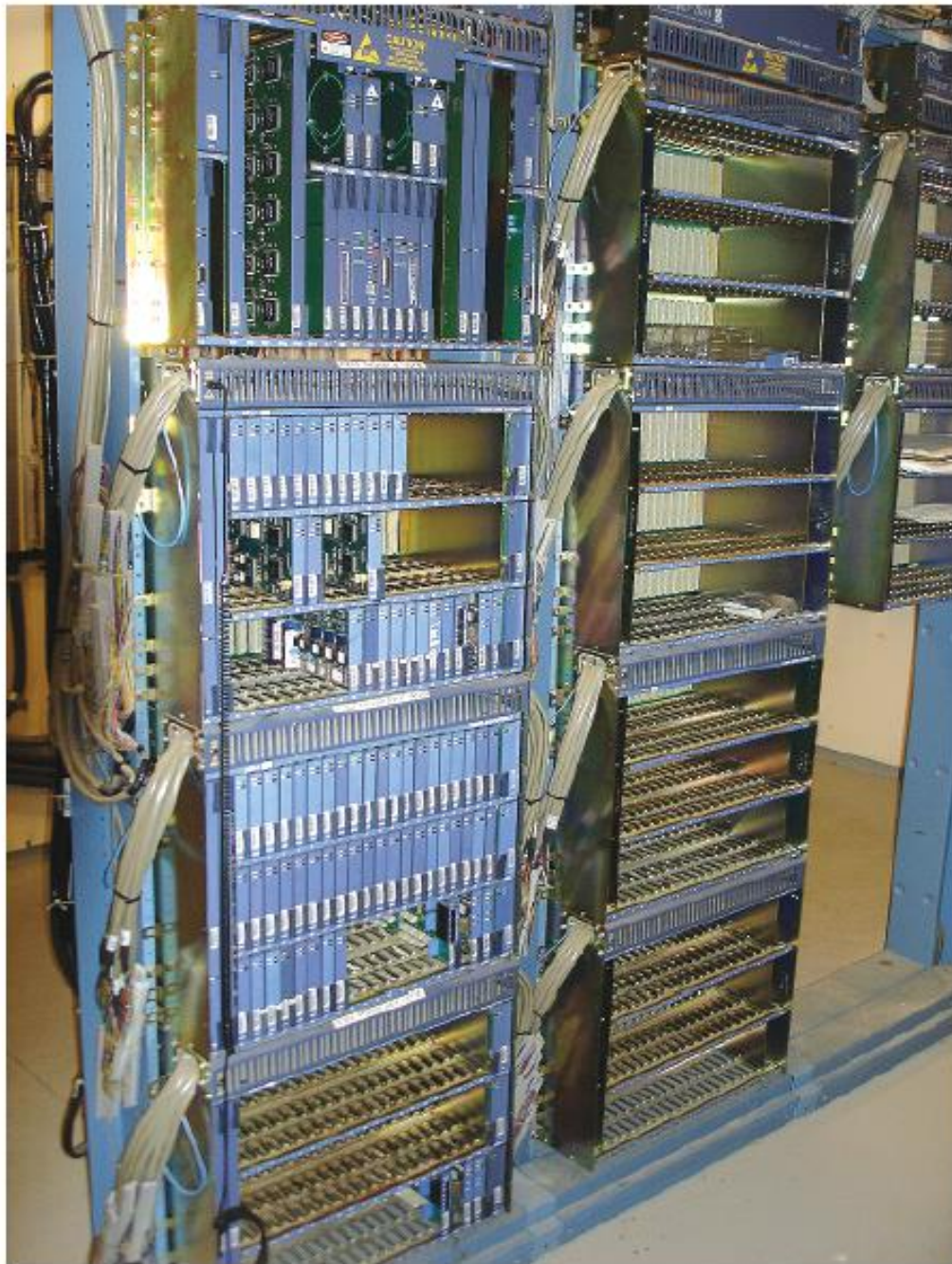
EXHIBIT 800.1 A private automatic branch exchange, one part of telecommunications equipment.
