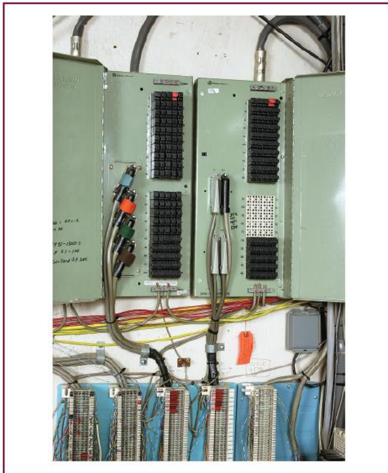
EXHIBIT 800.3 A primary protector unit installed in a commercial building that is the interface to the outside plant cable.
