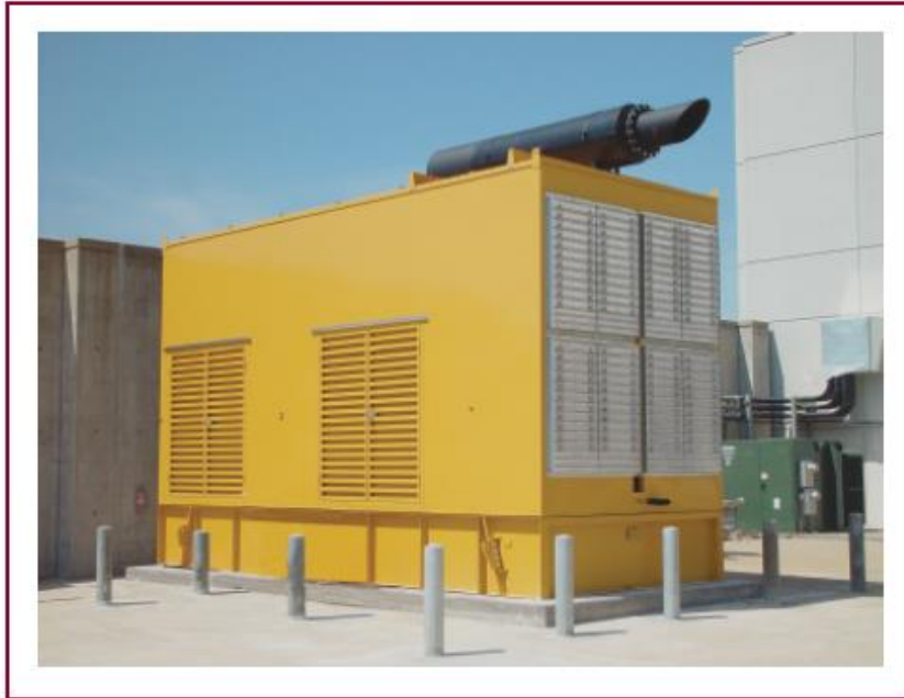
EXHIBIT 700.7 Alternate source of power in a heated and secure enclosure that is located in an area not subject to flooding. (Courtesy of the International Association of Electrical Inspectors)
