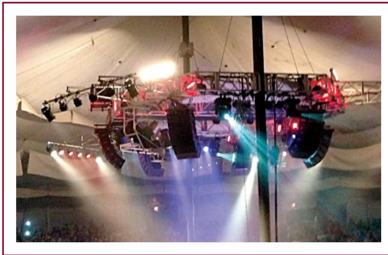
EXHIBIT 520.6 A suspended border light assembly over a stage.
