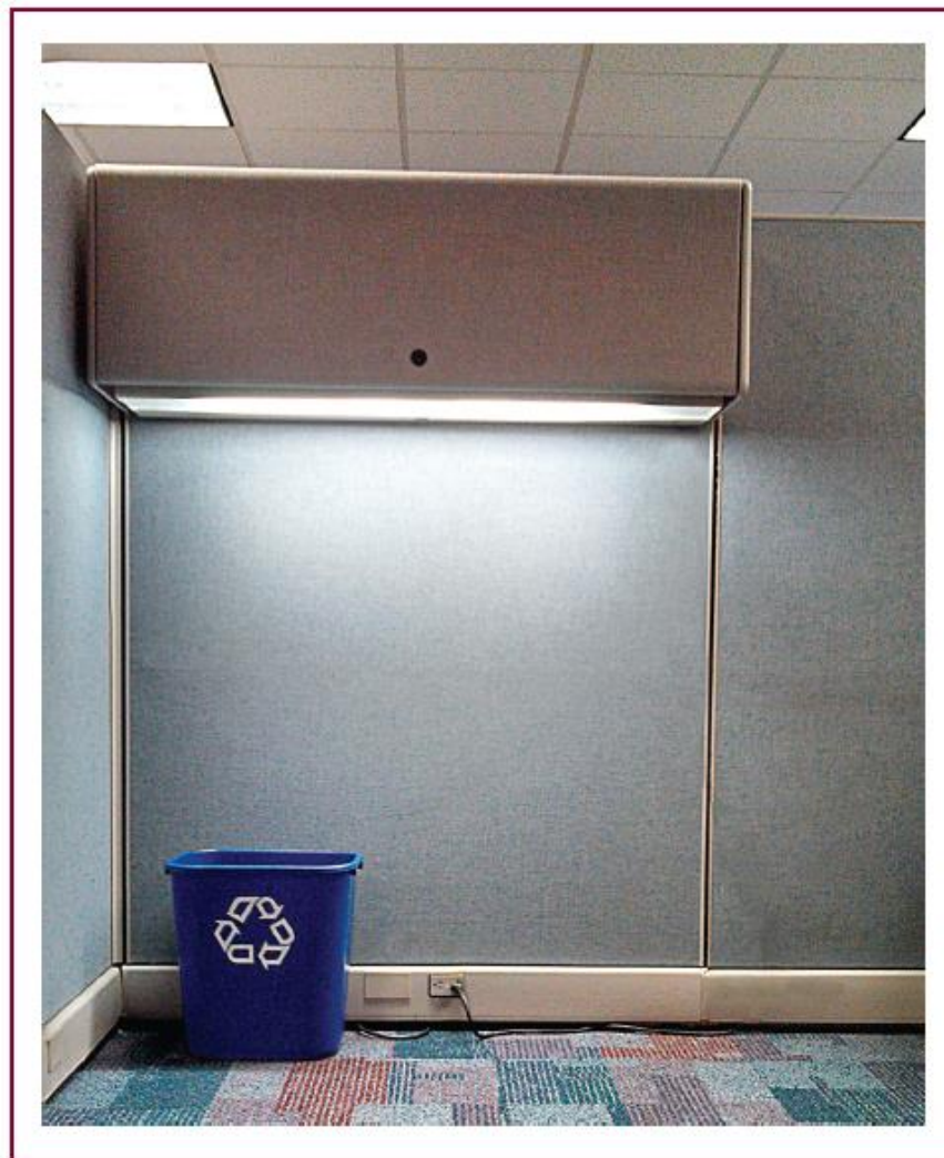
EXHIBIT 605.1 Example of a fixed-type office partition where the branch-circuit wiring is run through the partition.
