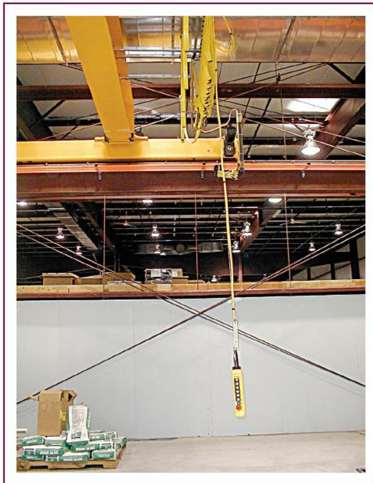
EXHIBIT 610.2 A suitable strain relief grip for a cord-suspended pushbutton station.
