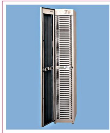
EXHIBIT 520.3 A typical high-density digital SCR dimmer switchboard. (Courtesy of Electronic Theatre Controls, Inc.)
