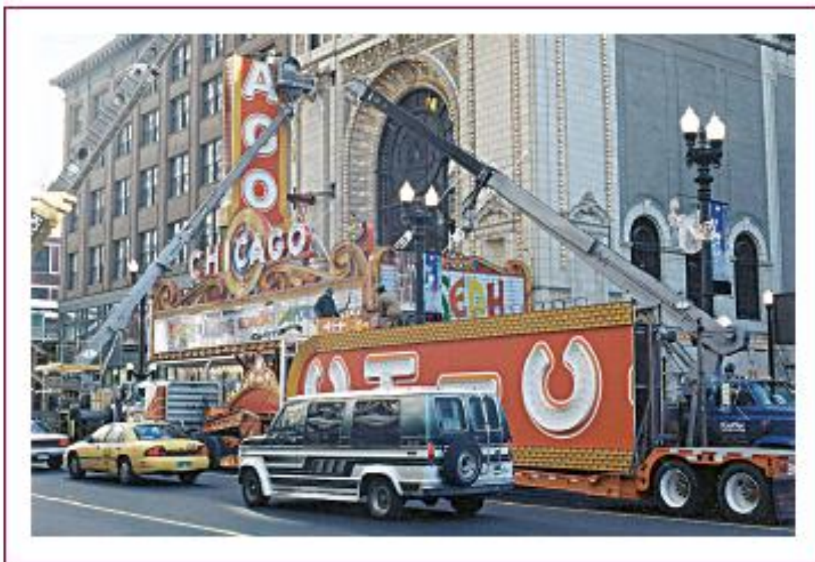
EXHIBIT 600.1 Example of a section sign where the subassemblies are field assembled to form a single sign. (Courtesy of Kleffer & Co. Inc.)
